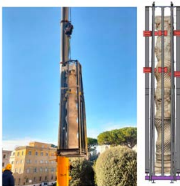
Figure 5 - The protection system of the Holy column during the transportation in the new room in the Vatican within the re-adaptation of the devotional spaces on the occasion of the Jubilee 2025
